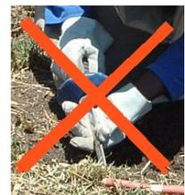
When the ground is too hard to use the Pick-prod effectively use the **SD Two-handed excavator** to break up the ground well back from the detector signal, then use the Pick-prod to loosen the face of the excavation.
